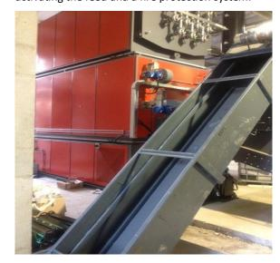
The wood chip fuel delivery reception and storage area is located in an above ground fuel store with moving floor hydraulic pusher device to feed fuel into the trough through a slot in the end wall. Due to restrictive access at the site, biomass is delivered to
