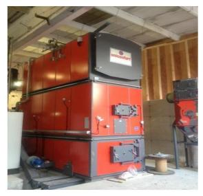
The feed system incorporates a cutting system for reducing oversize particles, min-max sensors for activating the feed and a fire protection system.
